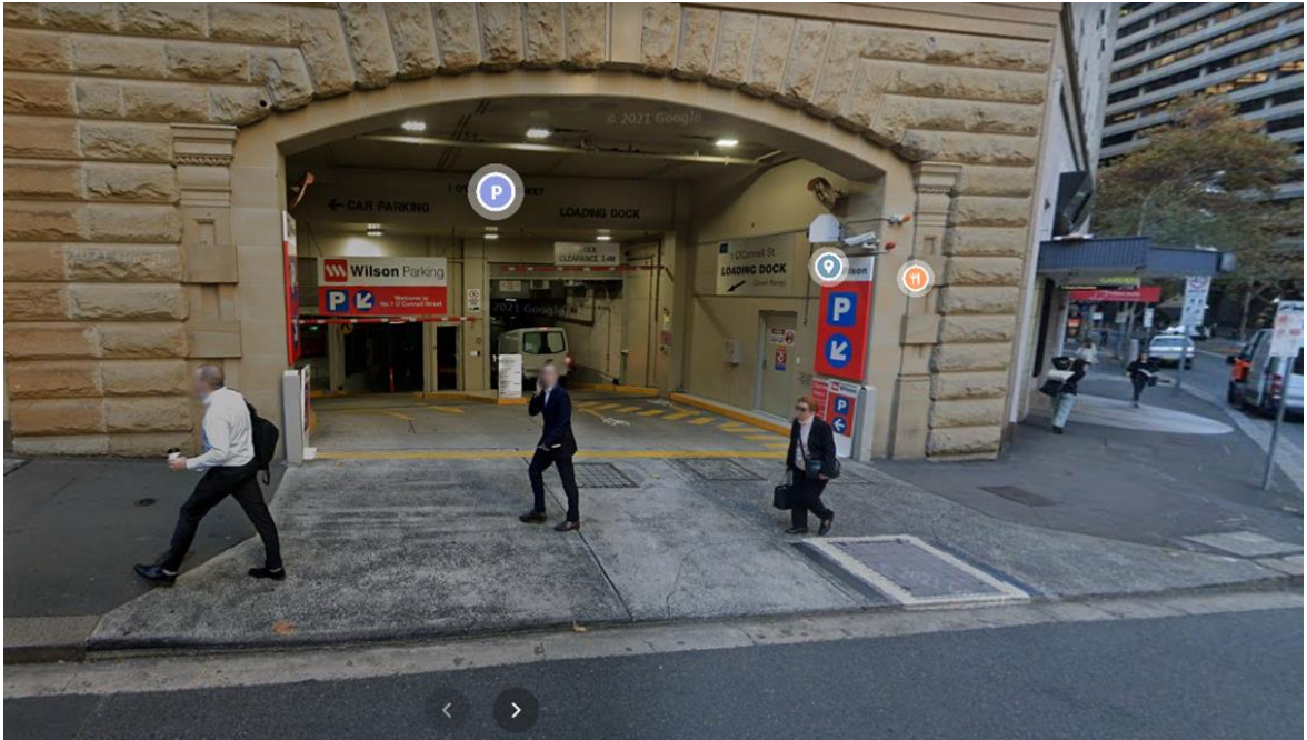
Figure 16 – Existing Bent Street Basement Car Park Entrance (Source: Google Streetview, 23 March 2022)
